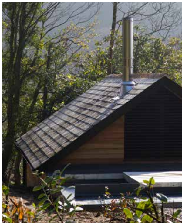
Wood chip boiler house, Restomel Manor
