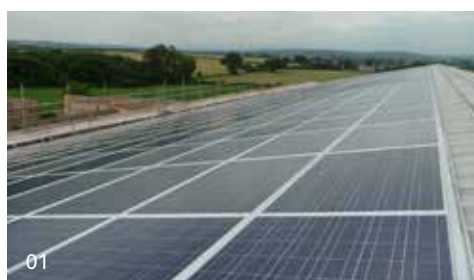
01. Farm building solar PV array, Hereford 02. Farm building solar PV array, Somerset
